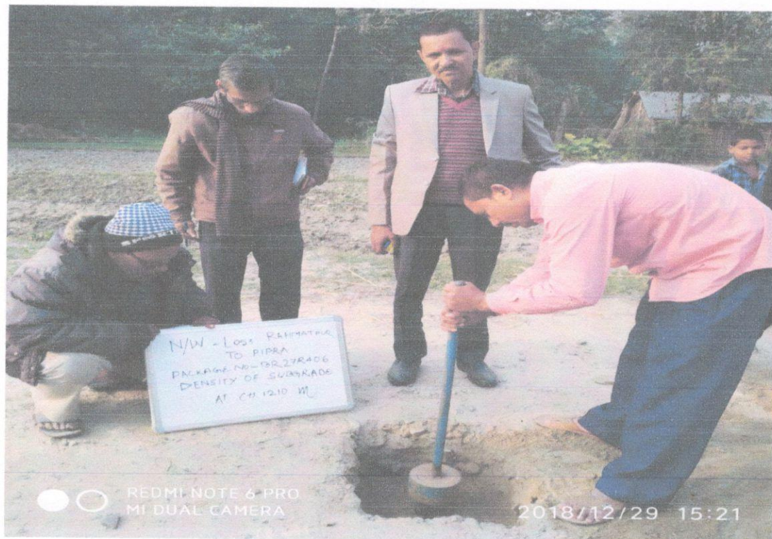
Density test of Sub-Grade at Km- 1/210
