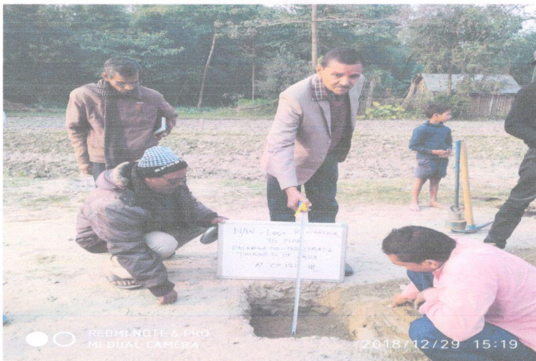
THICKNESS OF WBM GR-3+ gsb AT CH – 1/210 KM
