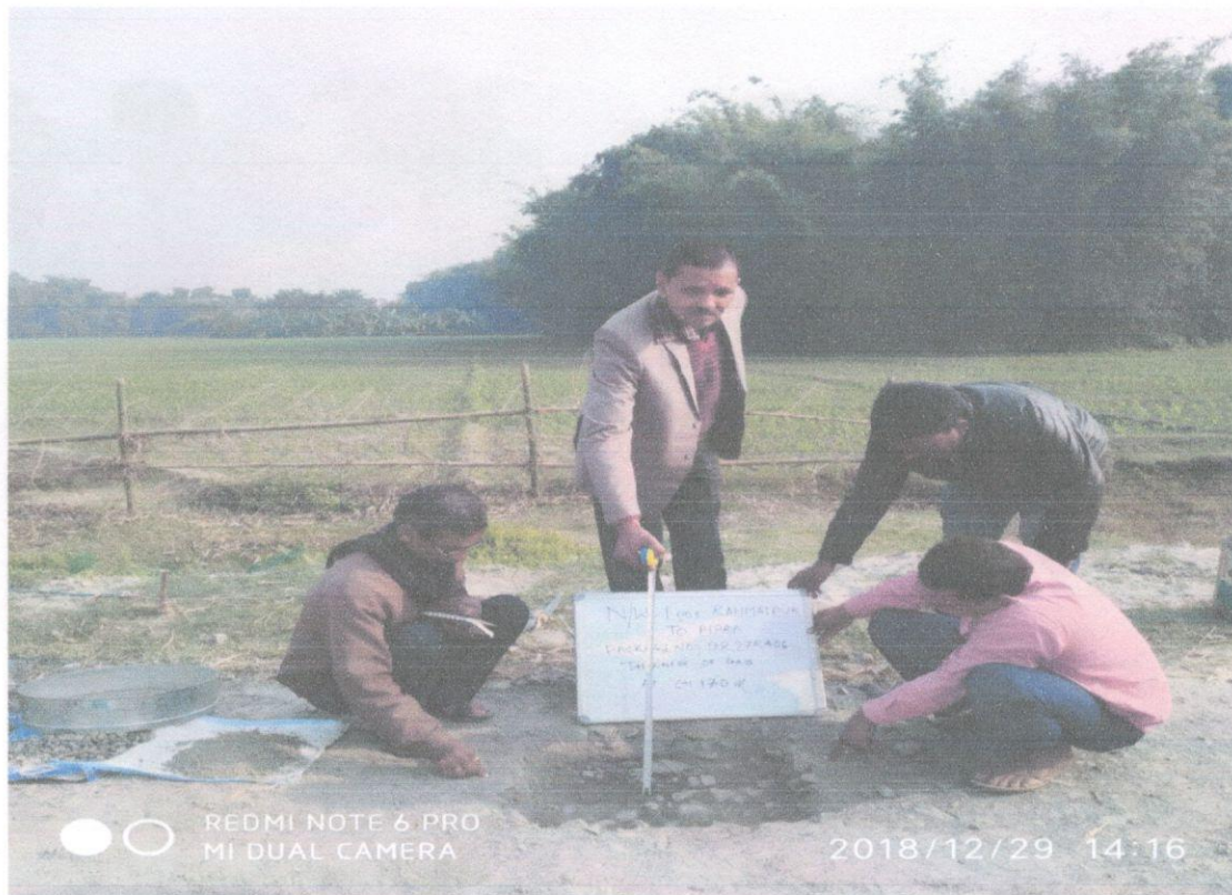
THICKNESS OF WBM GR-3 AT CH – 0/170 KM
