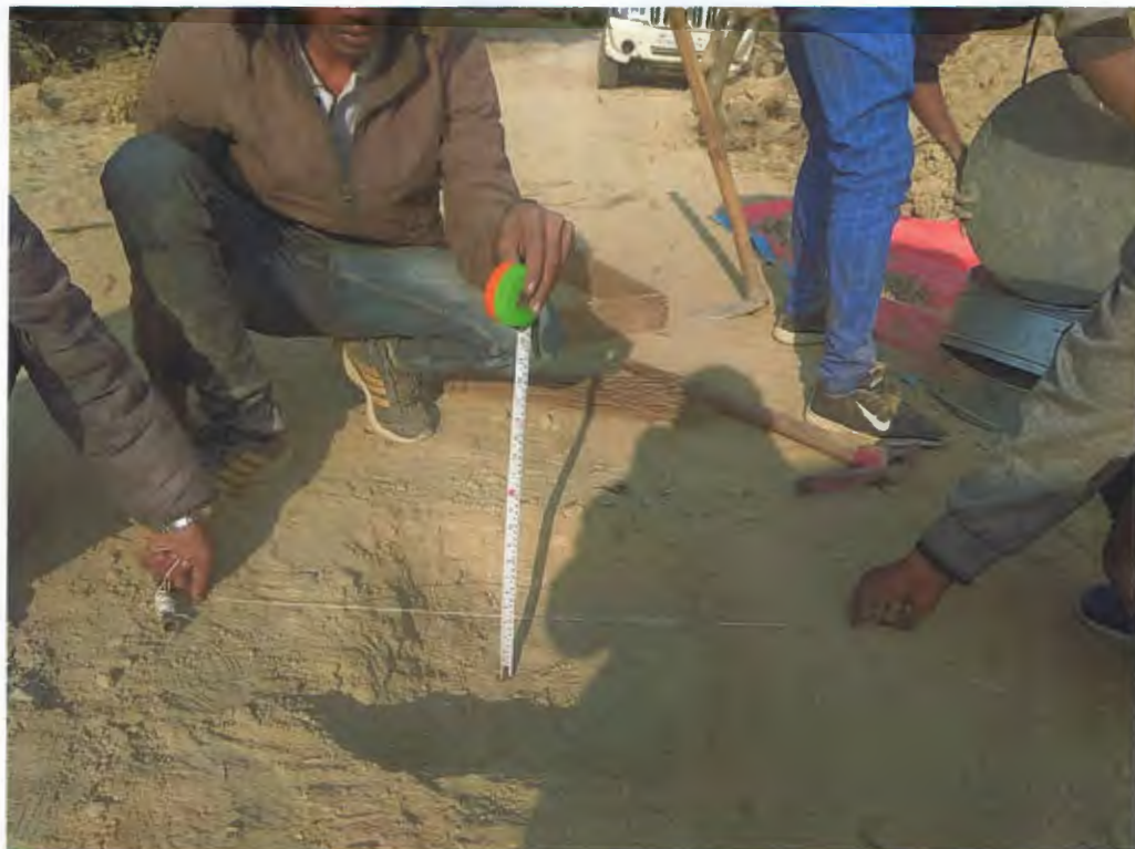
Thickness test G.S.B. at CH- 1.10 K.M.
