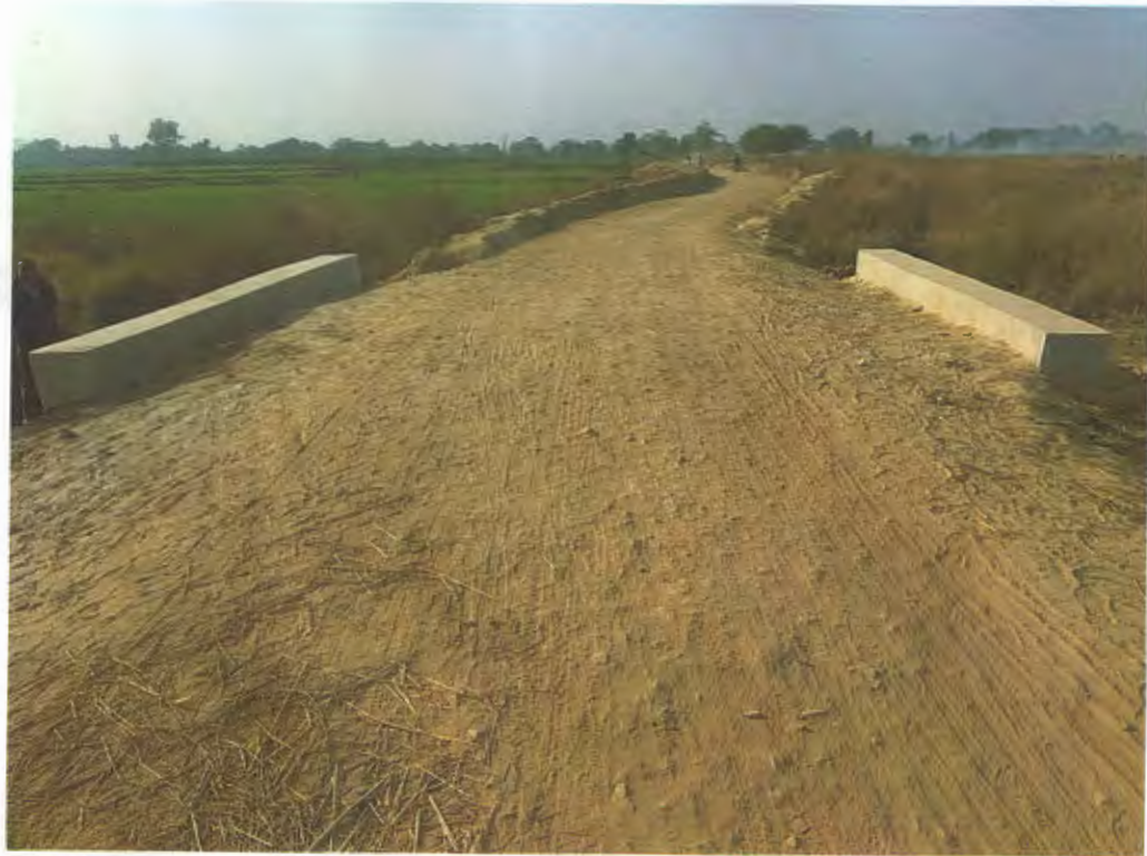
General view of road at CH- 0.00 K.M.
