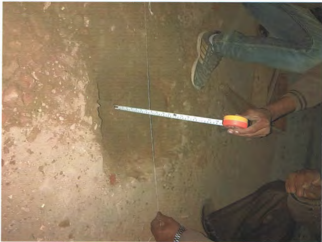
Thickness test of WBM-Gr II, Gr III at CH- 0.750 K.M.
