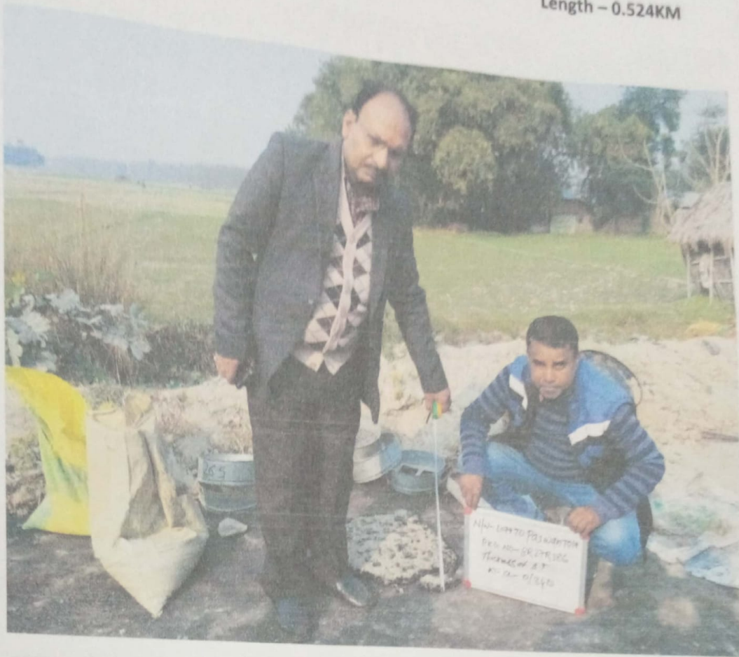
THICKNESS OF B T AT CH- 0/200
