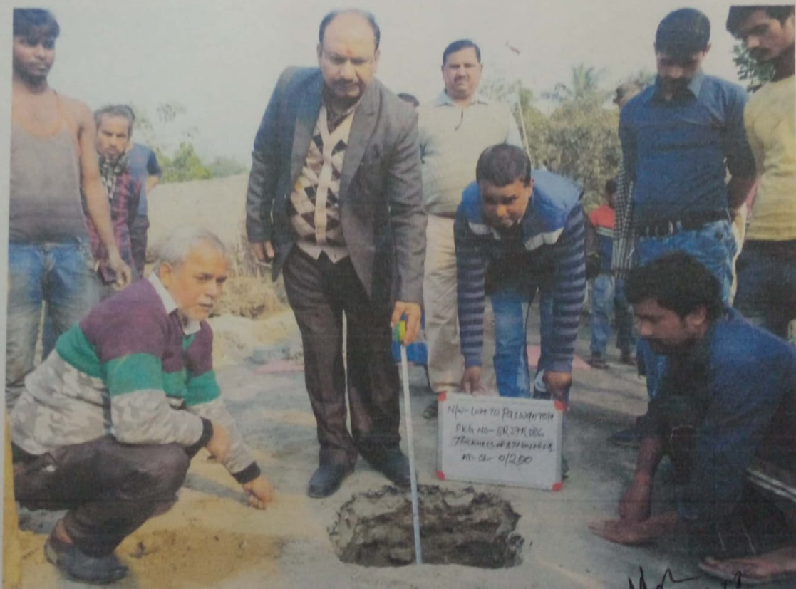
THICKNESS OF B T+ WBM GR-3 + GSB AT CH - 0/200
