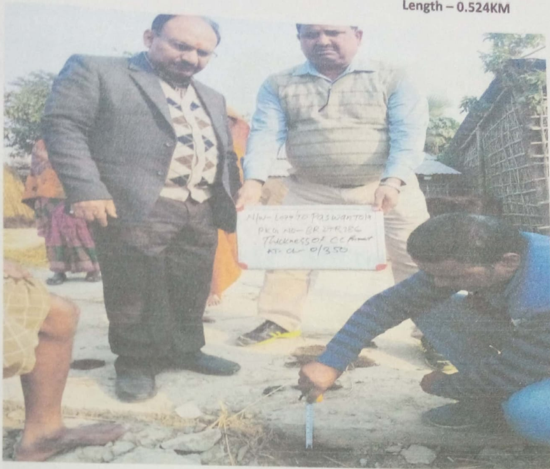
THICKNESS OF C C PAVMENT – 0/350
