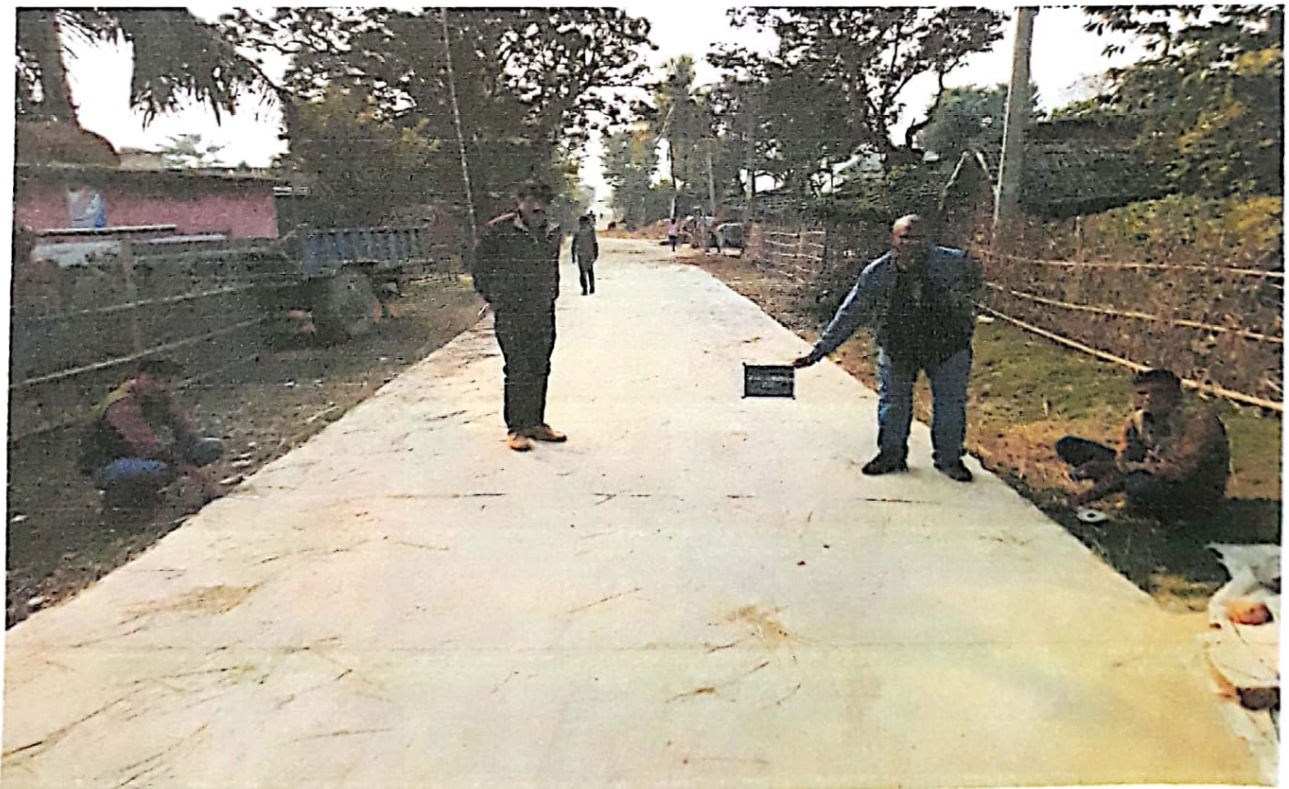
C/KI and GEN. VIEW OF C.C. PAVEMENT AT CH 325M
