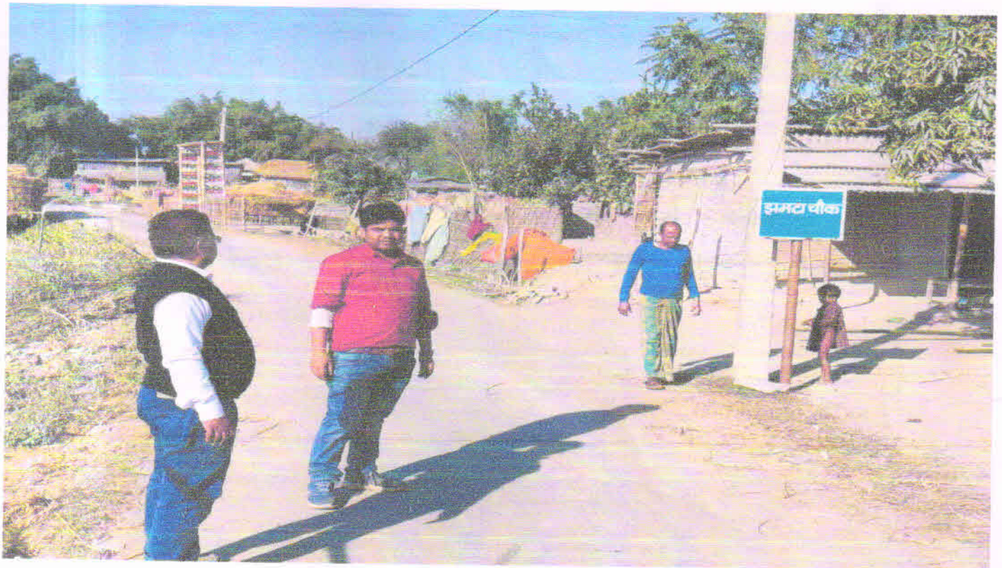
GENERAL VIEW OF ROAD AT CH - 1.750 K.M.
