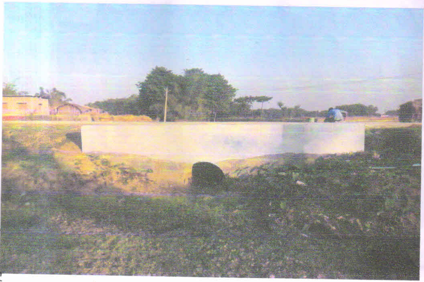
C.D. WORK AT CH = 100 M.
