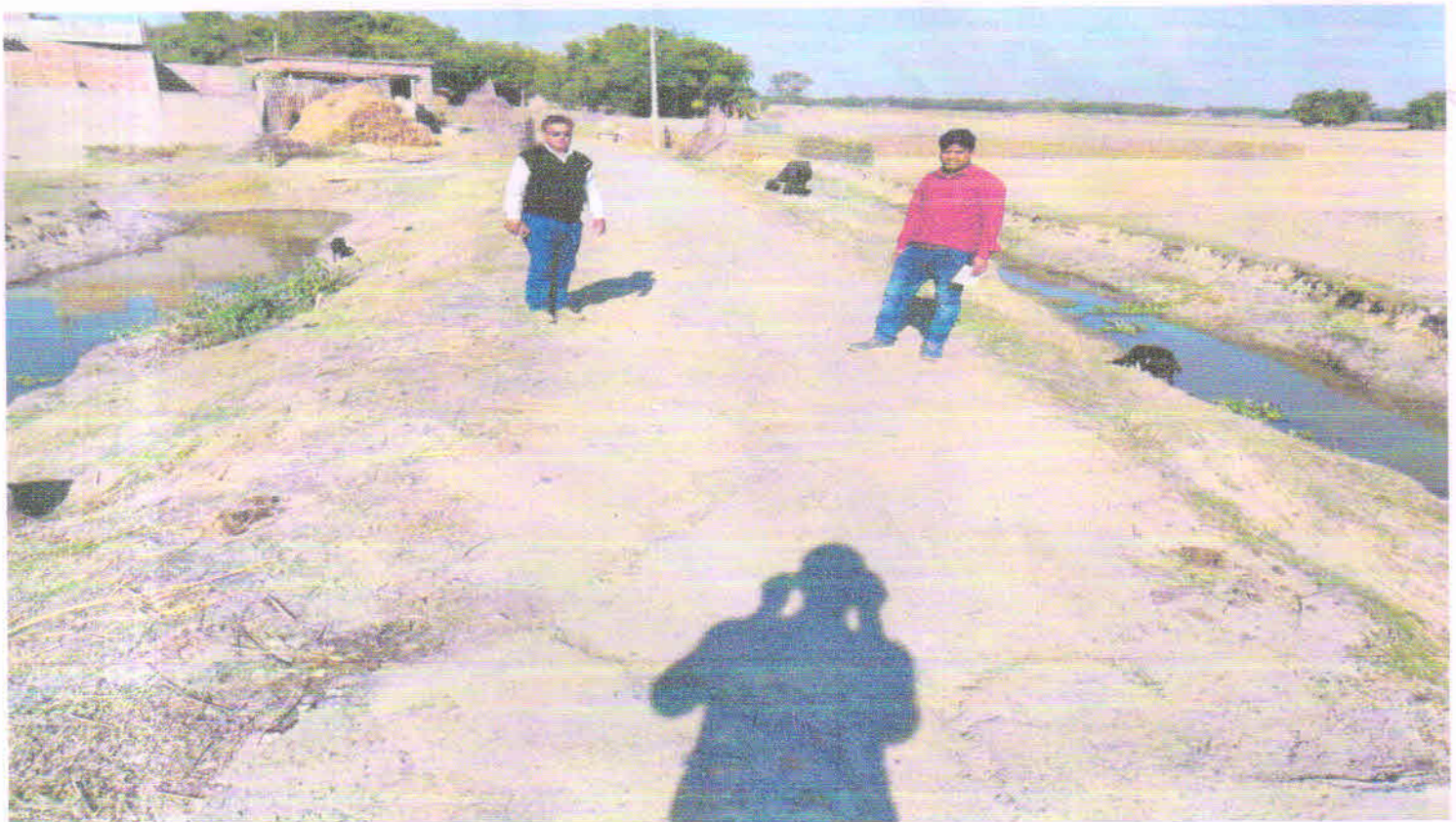
GENERAL VIEW OF ROAD AT CH=0.400 KM
