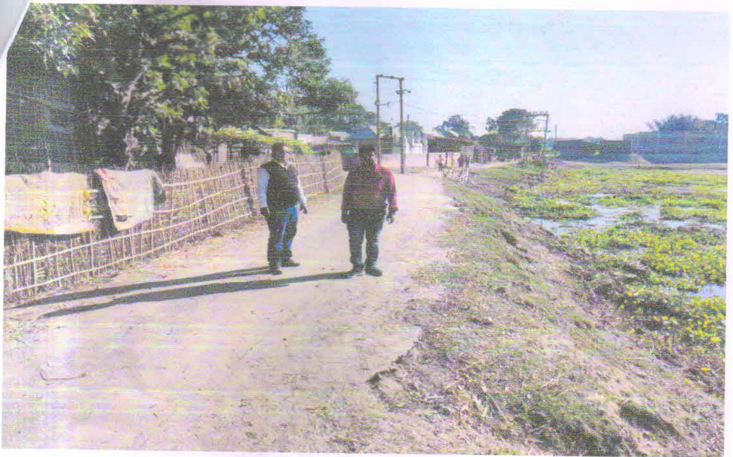
GENERAL VIEW OF ROAD AT CH - 1.600 K.M.
