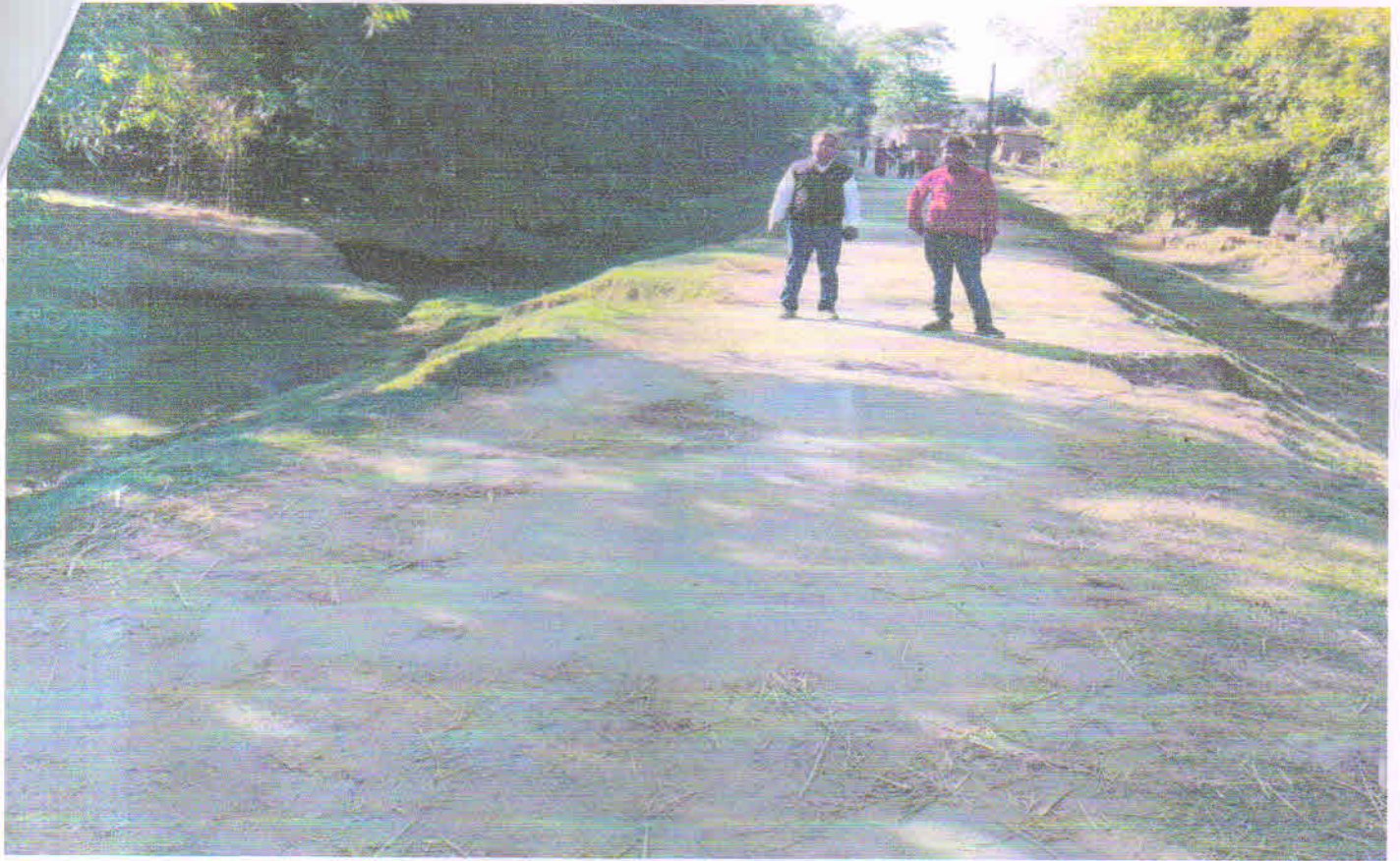
GENERAL VIEW OF ROAD ATCH - 1.100 K.M.
