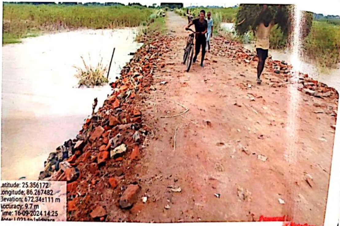
Filling of Brick bat after 1 st spell of flood
