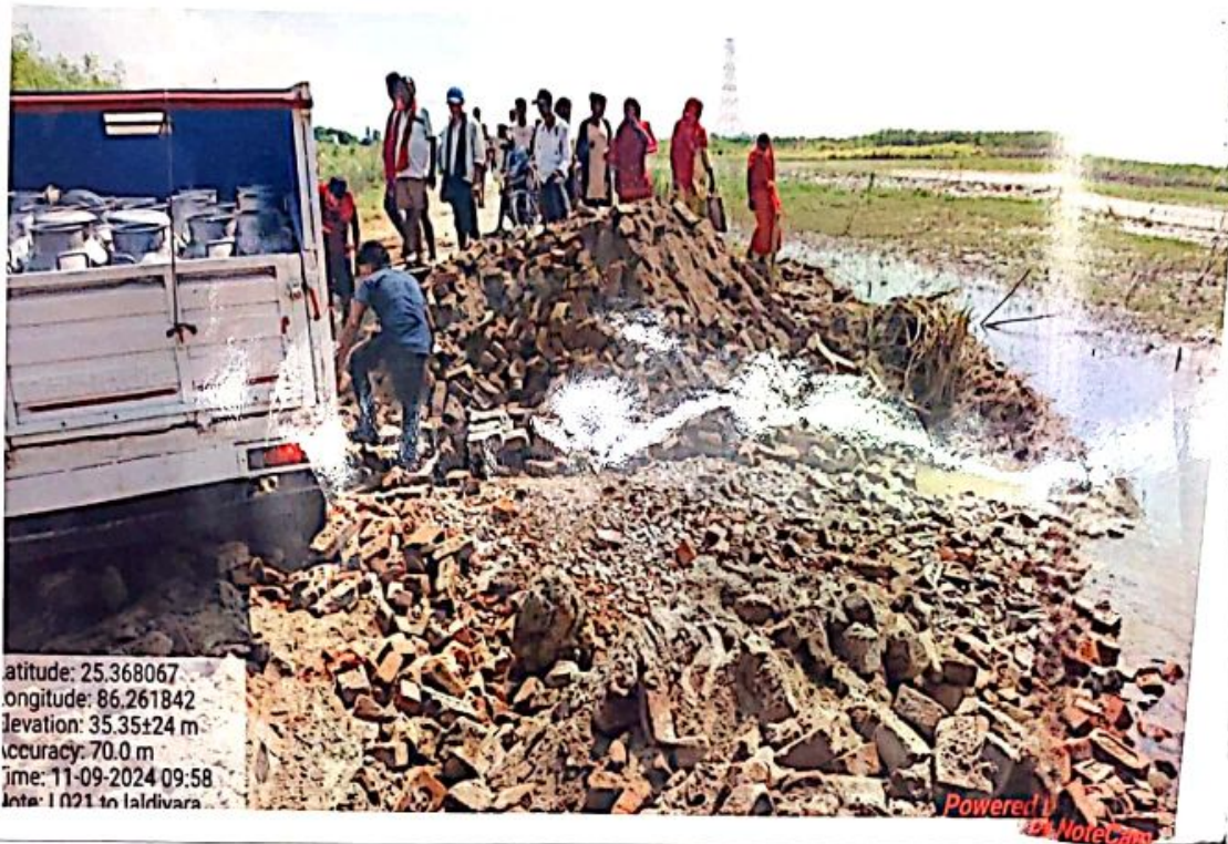
During filling of brick bat after 1 st spell of flood
