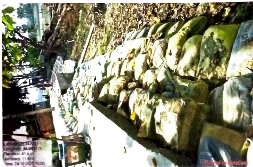
General View of Repaired Road
