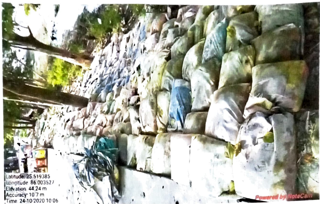
General View of Repaired Road
