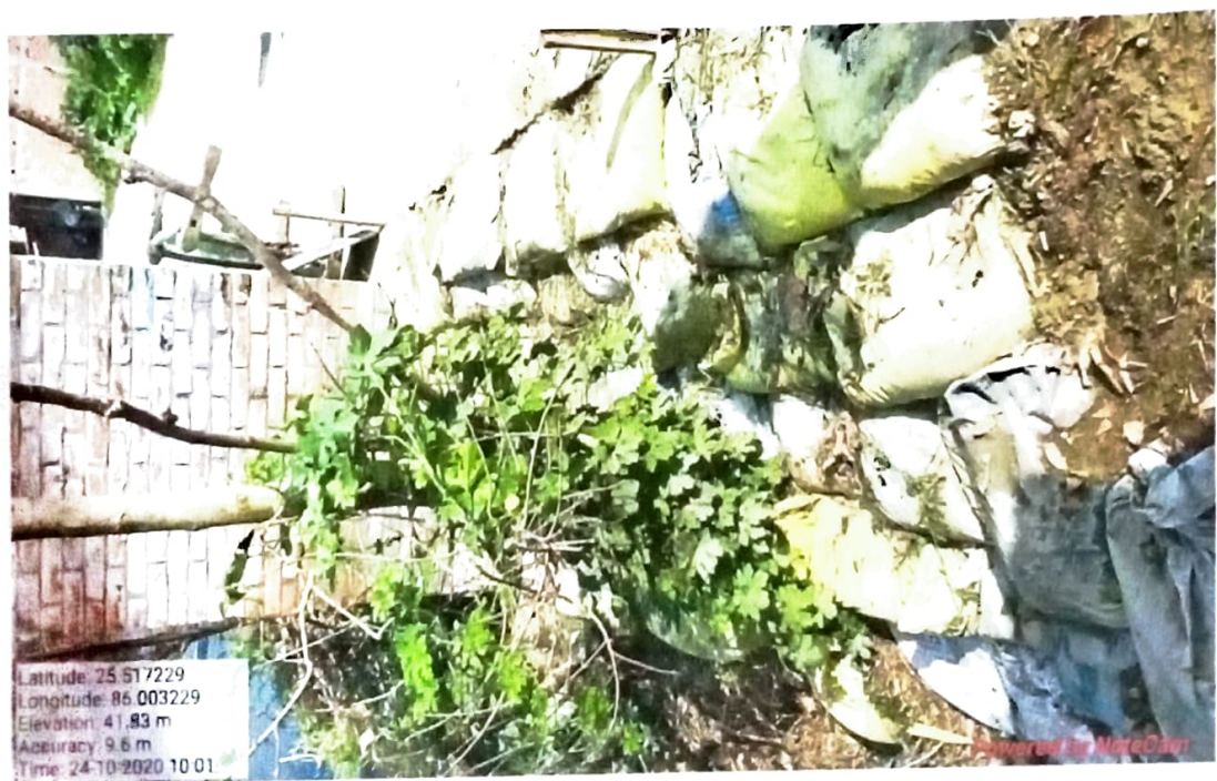
General View of Repaired Road
