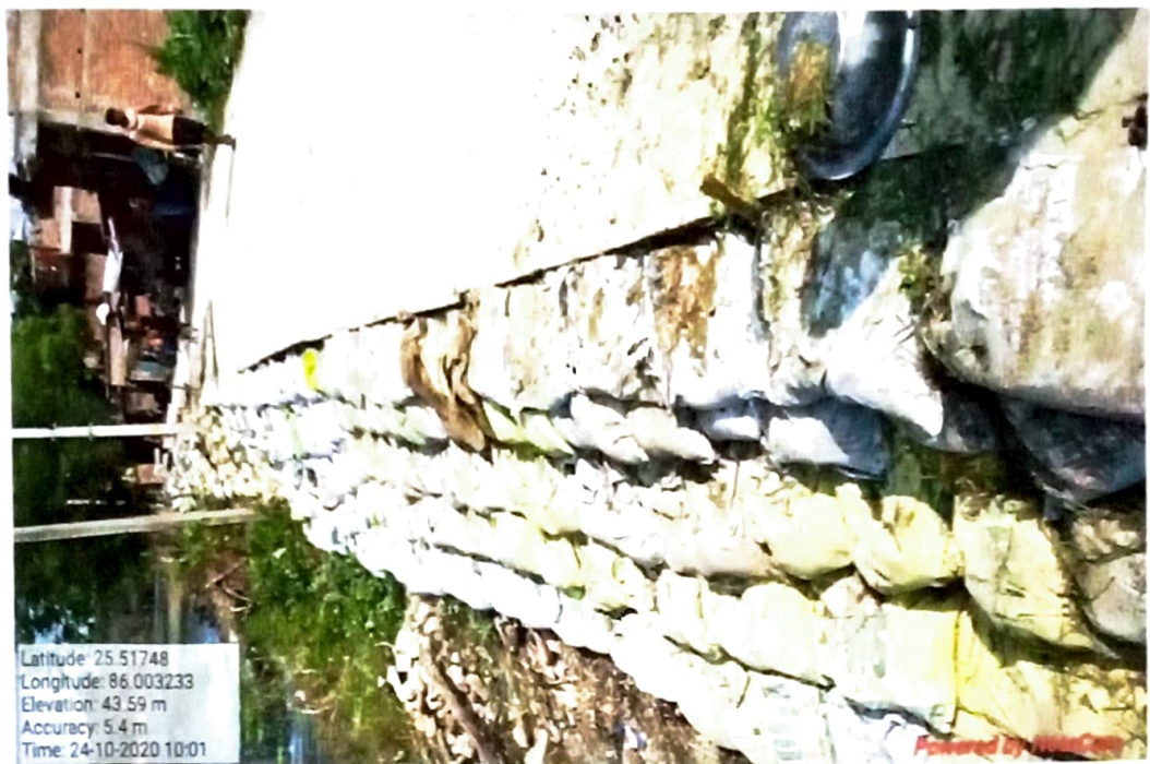
General View of Repaired Road
