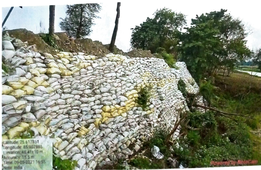
General View of Repaired Road
