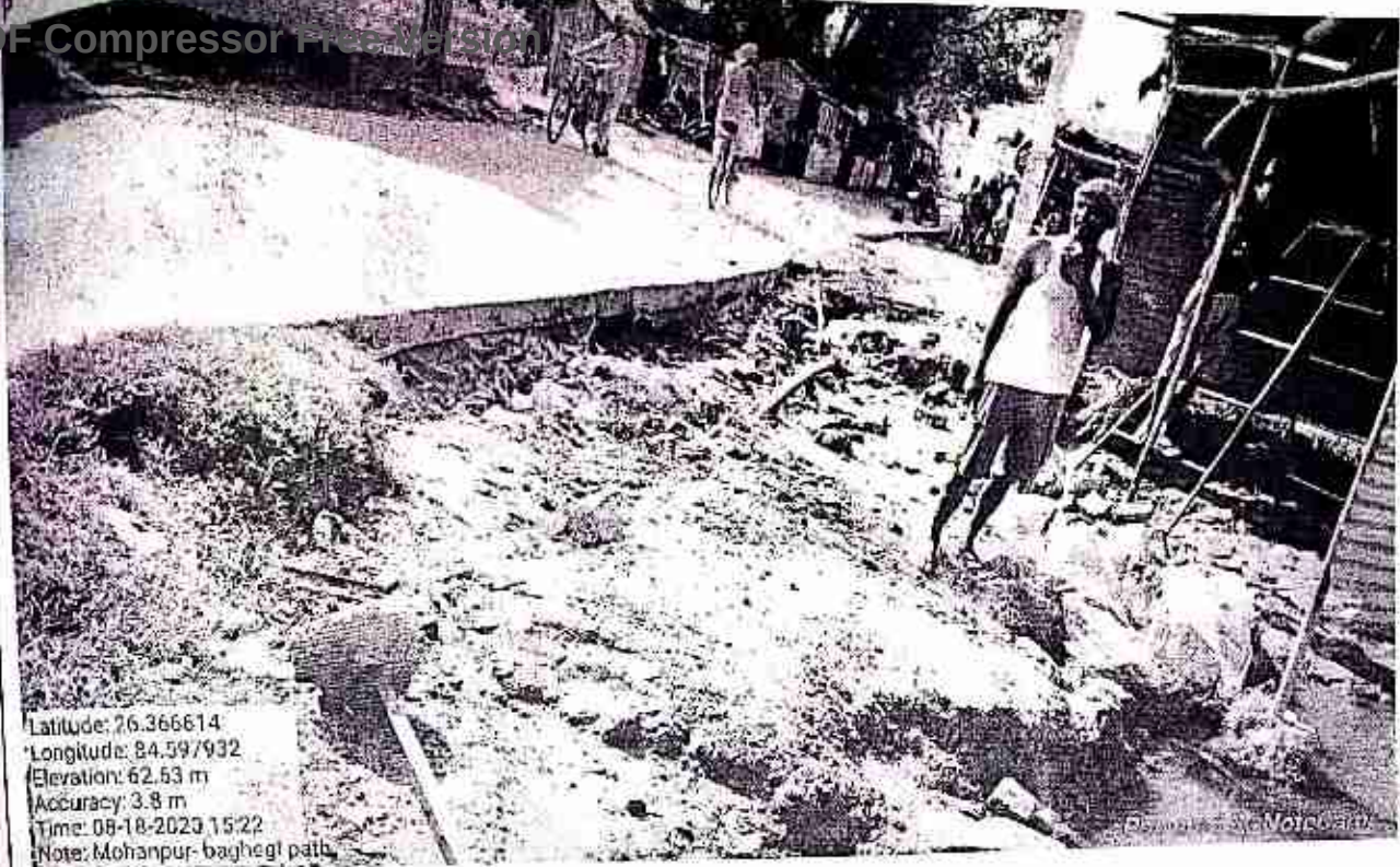
Motorable work of Mohanpur to Bagheji Road
