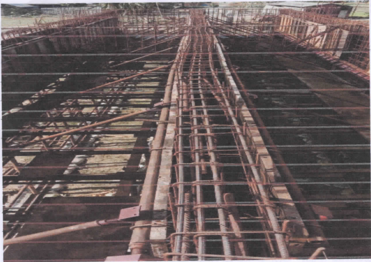
Const. of HL Bridge over Kanki River in 2 nd Km of Hublidangi To Ichamari Road Under – NABARD
